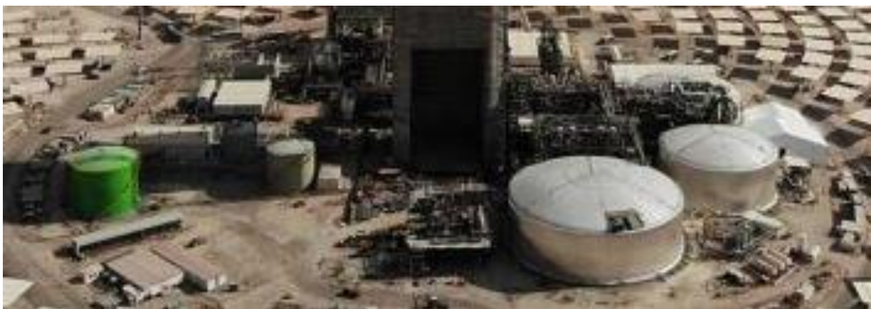
Figure 2: 17hour 110MWe molten salt storage system at CSP tower project Cerro Dominador in Chile (14)
